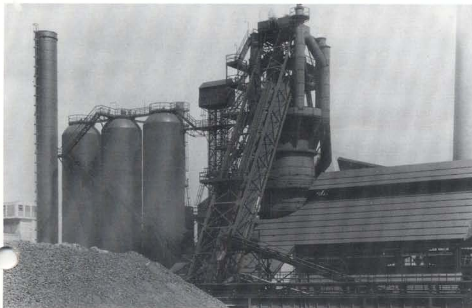
This photograph shows the blast-furnace and Cowper hot-blast stoves, which once dominated Ford's Dagenham factory site.
