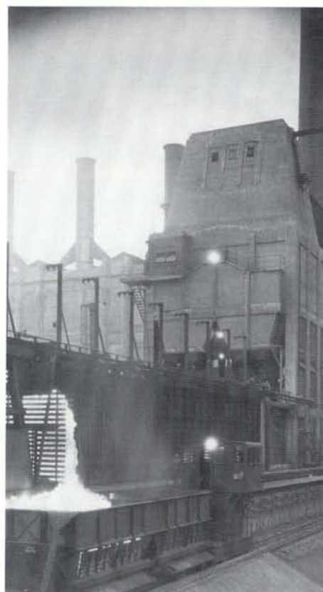
The coke ovens on the Ford site at Dagenham provided fuel for the blast-furnace.
